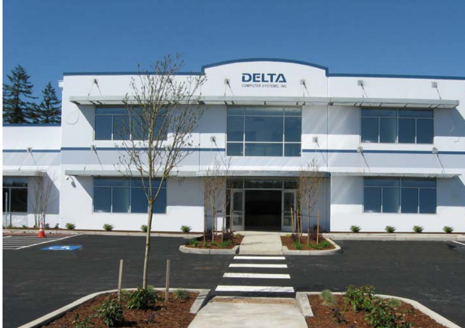
Caption: DELTA's new Battle Ground WA headquarters building
